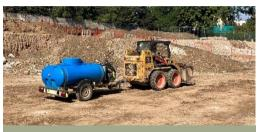
Water tankers transport water to dust suppression systems around the site.
