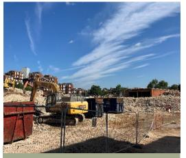
Demolition materials being separated for reuse and recycling.
