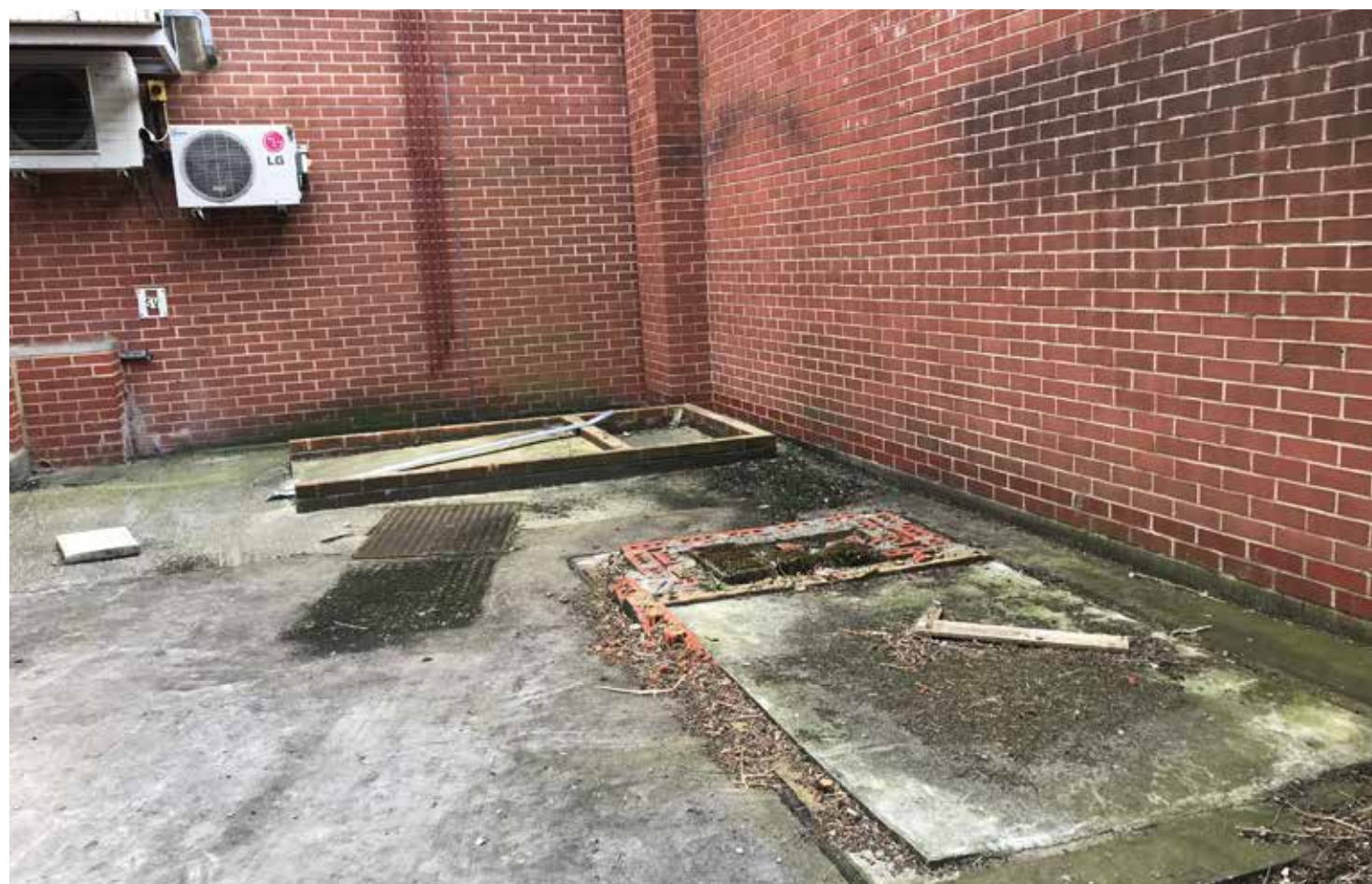
Concrete plints in central area of the Site.
