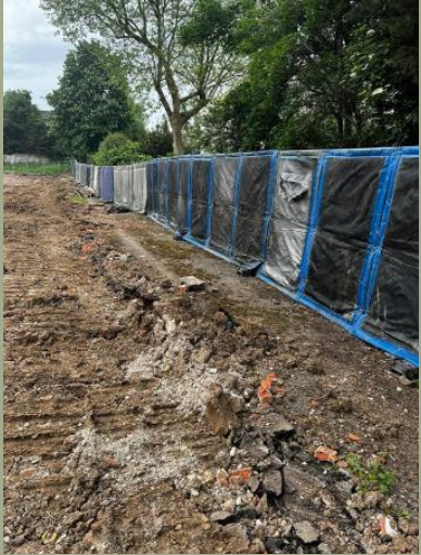
Noise reducing blankets used along the hoarding line.
