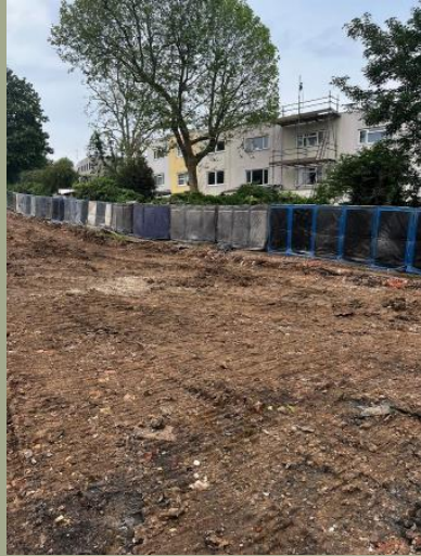
Noise reducing blankets used along the hoarding line.
