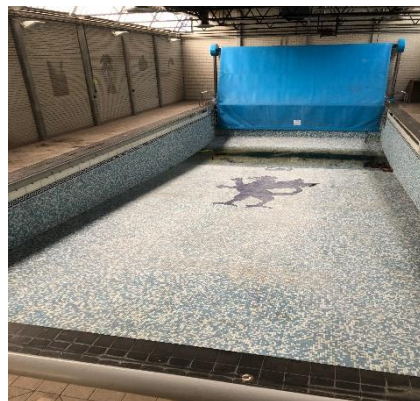
Former swimming pool
