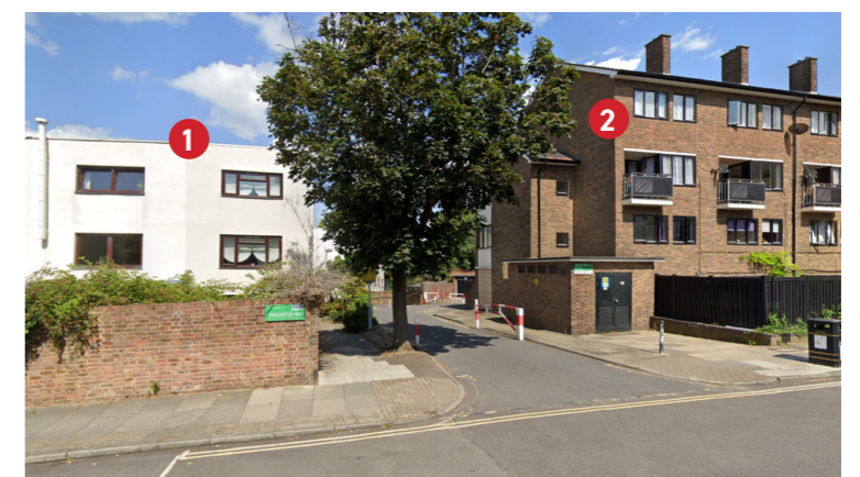
View from Dalmeny Ave, existing storage
