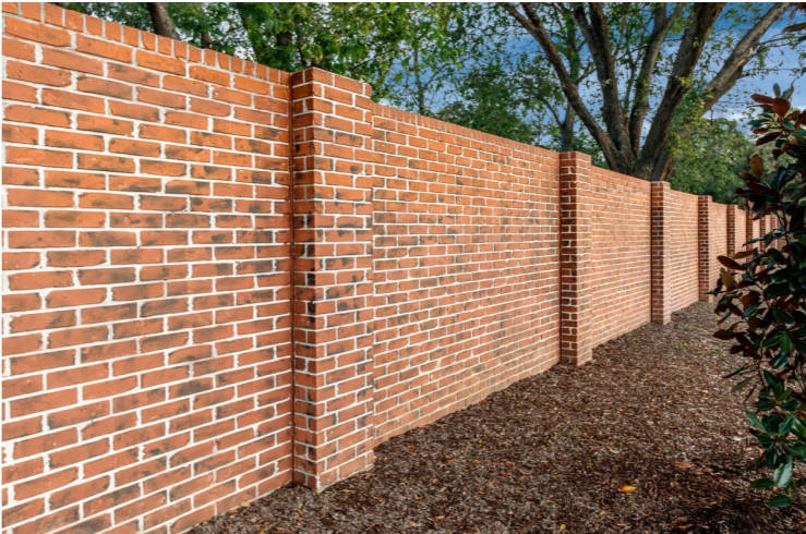
BRICK WALL - 1.8M HIGH
