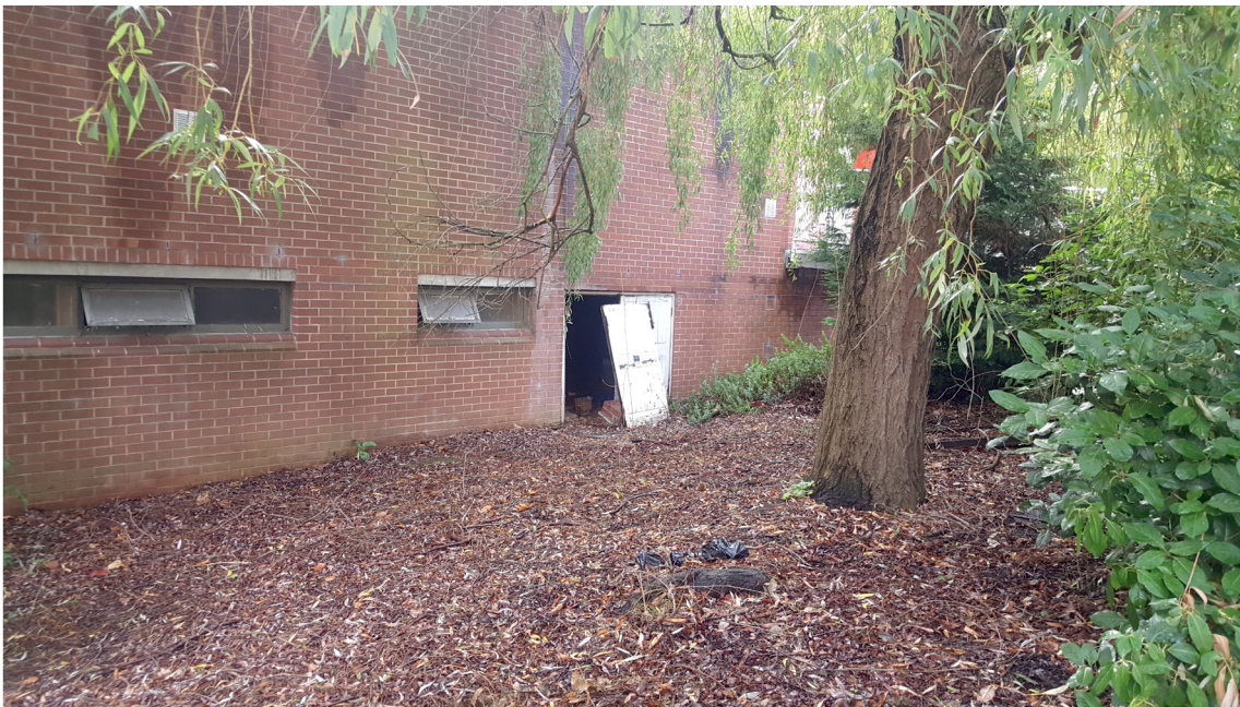
Fig 16 Photograph of Holloway Prison building cutting into existing ground level (MOLA 2019)
