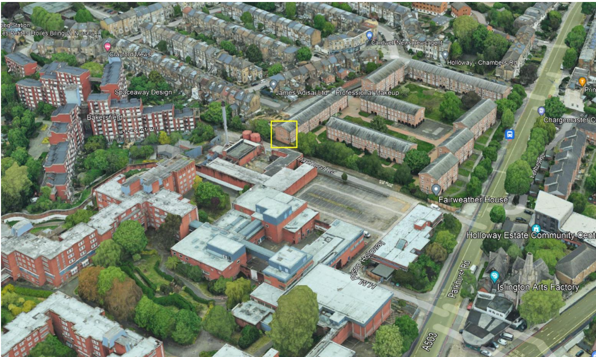
Figure 23: Aerial image showing location of noise sensitive receptor used in example plant noise emissions calculation
