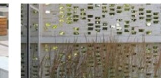
BREEZE BLOCK WALL
