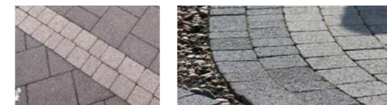
Surface Type 07 CONCRETE SETTS To memory garden, cycle parking areas and smaller static spaces
