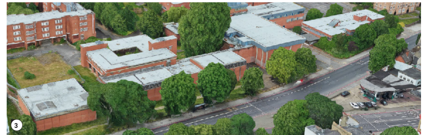
View of Camden/Parkhurst Road and the existing mature trees that line the streetscape.
