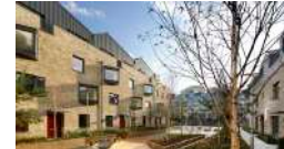
Wharf Road, Angel
