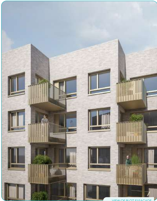
VIEW OF PLOT E1 FACADE
