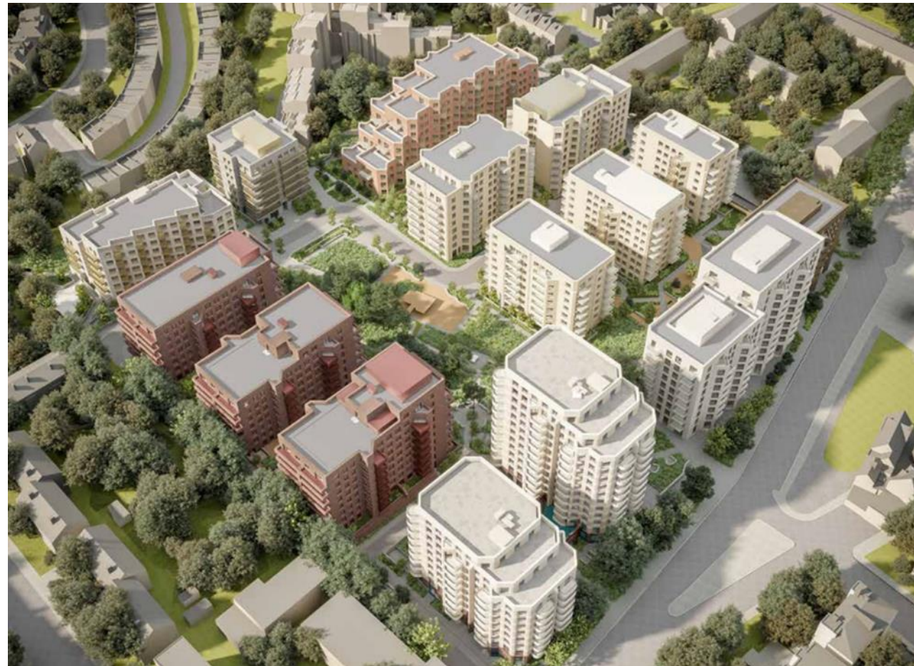
Figure 1 - Site Image (Credit: AHMM)
