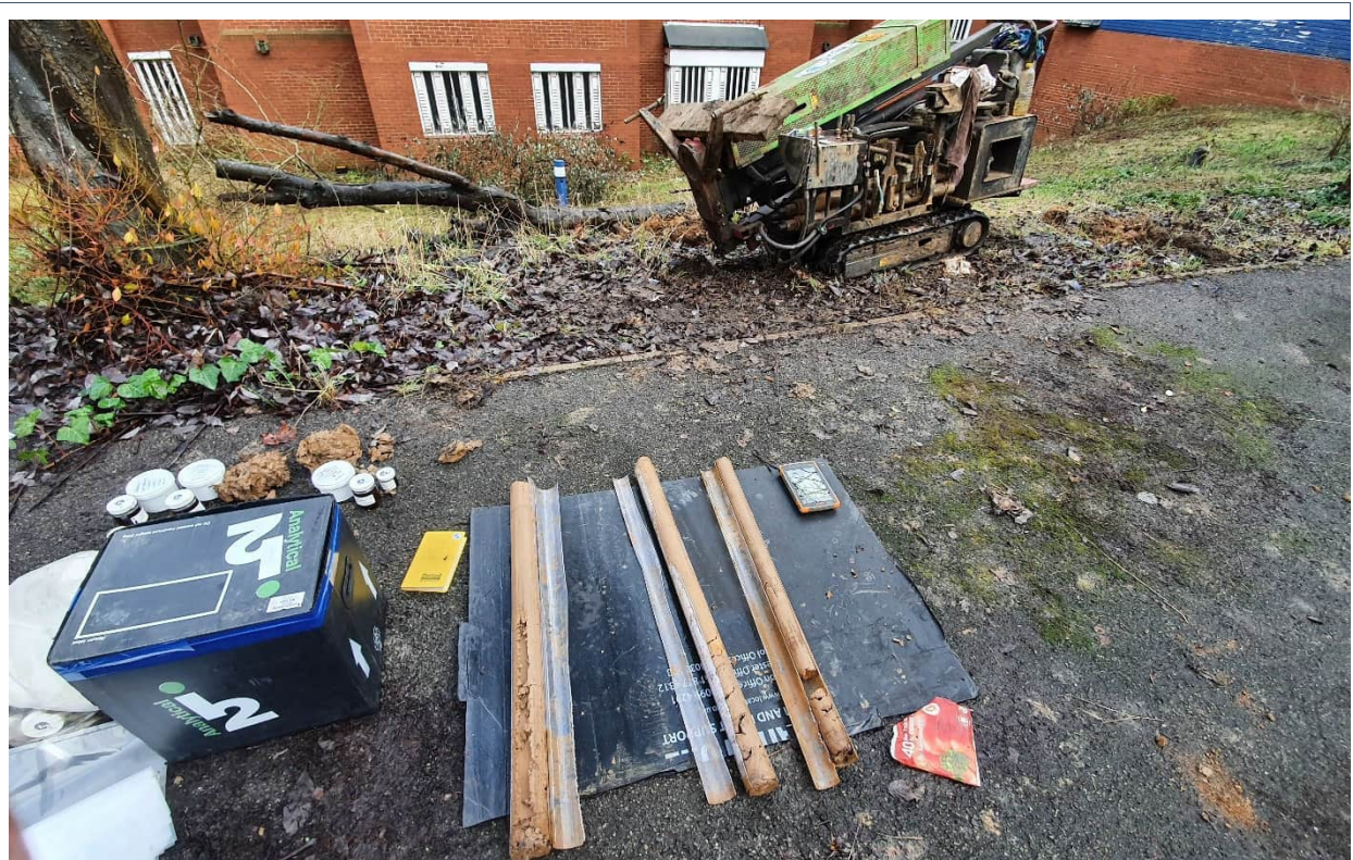
Photograph 4 - Window sample rig in position over WS02.
