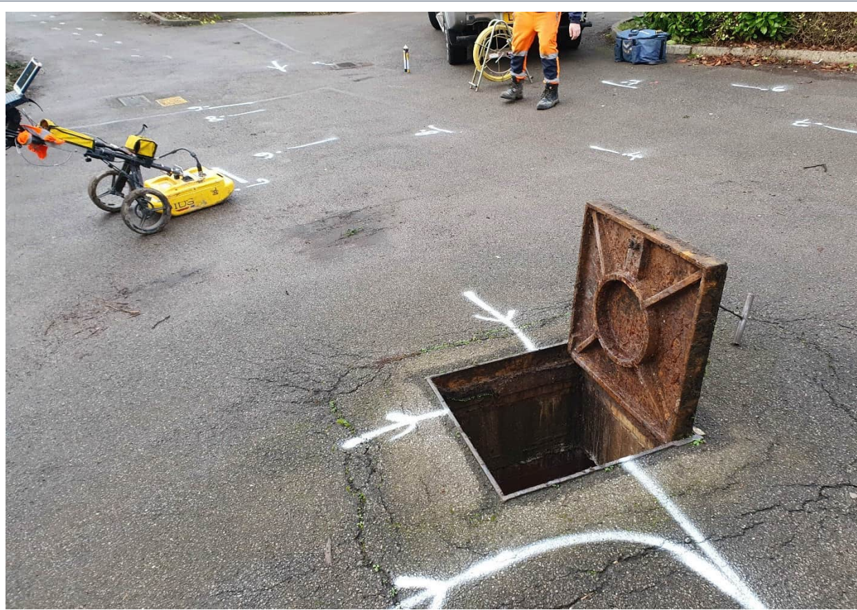
Photograph 1 – Utilities Clearance being undertaken at the proposed location of BH14.
