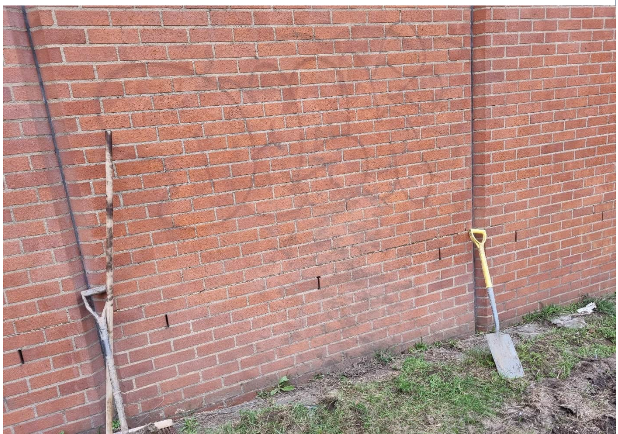
Photograph 14 – Wall by BH15 post cleaning up.
