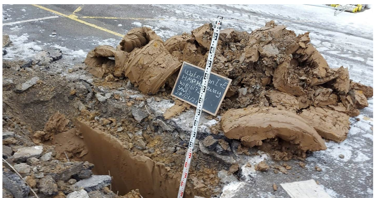
Photograph 5 – SA01 before the soakaway test was undertaken.
