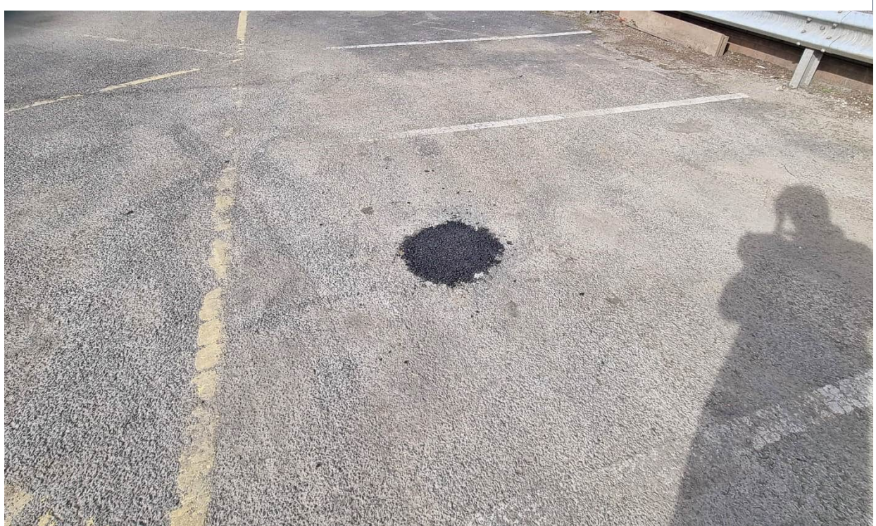
Photograph 13 – BH03 post reinstatement.
