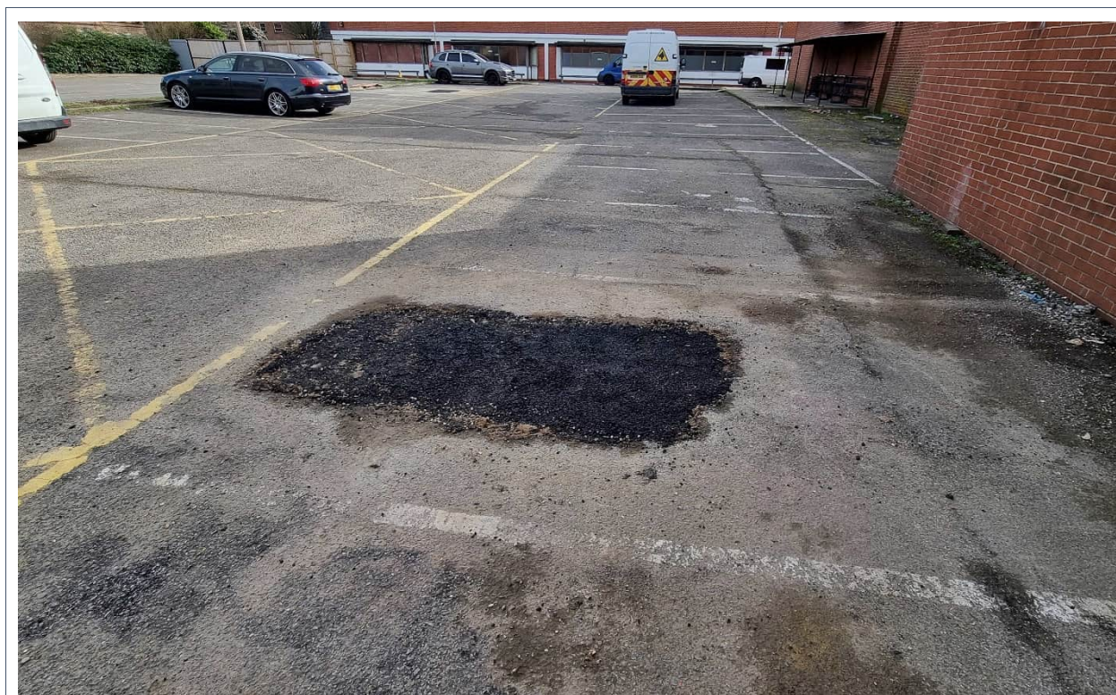
Photograph 11 – TP05 post reinstatement.
