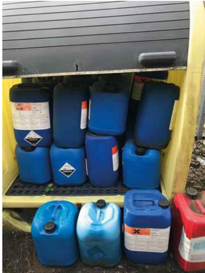
Contents of yellow bund, including acid, water treatment chemicals and herbicides.
