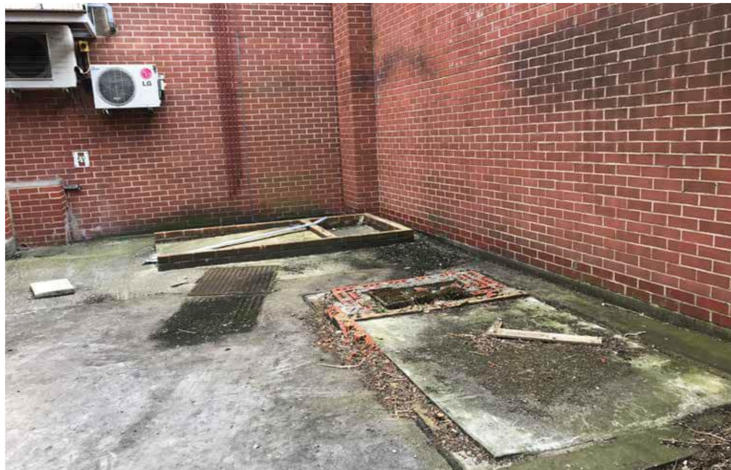
Concrete plinths in central area of the Site.
