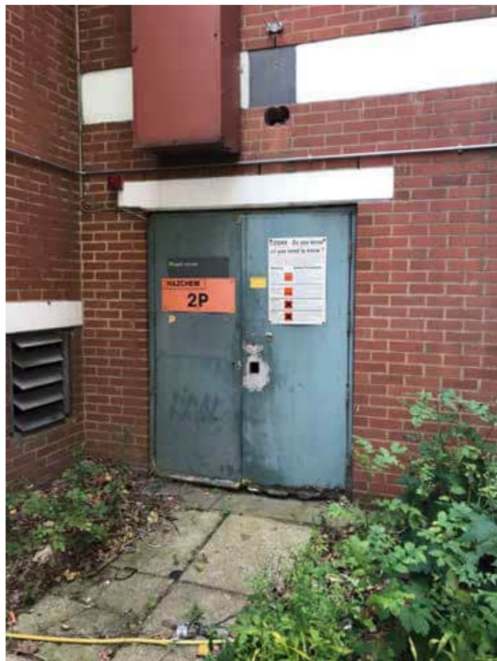
Plant room in the southeast of the Site.
