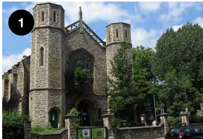
1 Camden Road Baptist Church
