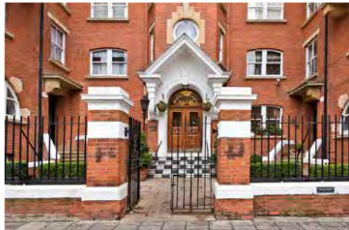
Moscow Road Mansions, Bayswater
