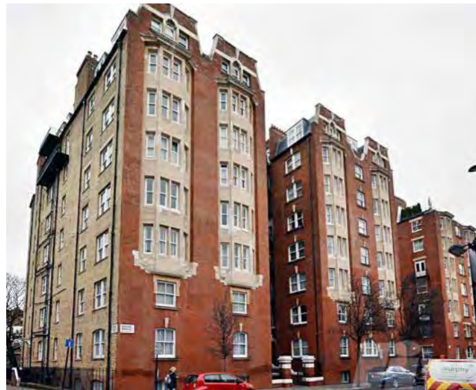
Moscow Road Mansions, Bayswater
