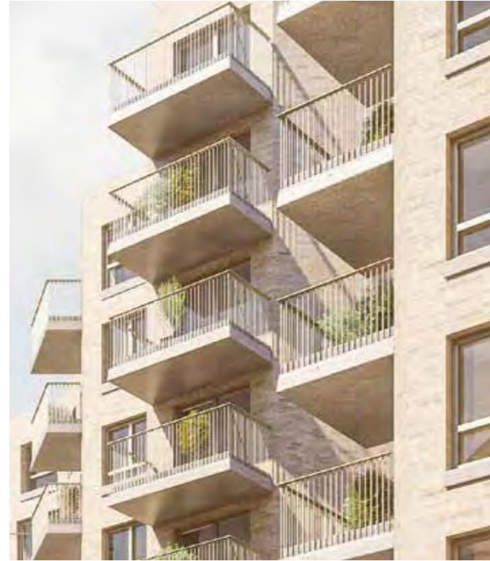
● Concrete balconies with metal guarding and handrail
