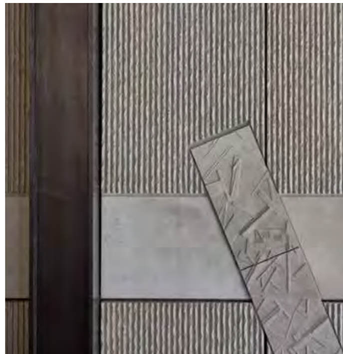
Example of cast concrete wall relief Soho Place by AHMM for Derwent London Artist: Marcin Dudek
