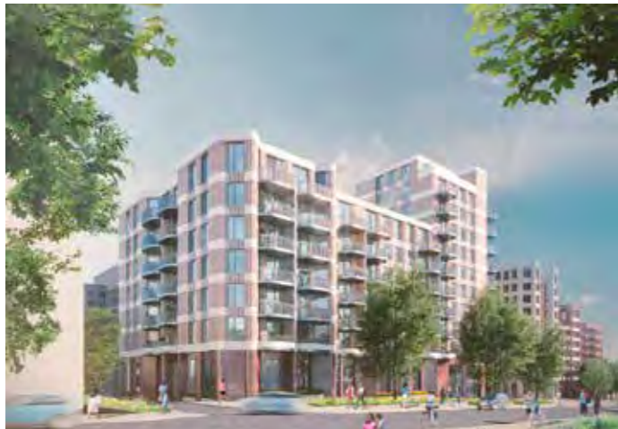
View looking north-east from Camden Road
